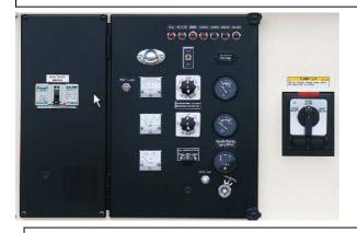
Engine operating switch behind control panel
