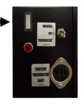
ATTENTION: IF RED LIGHT IS INDICATED, MAKE CORRECTIONS TO POWER SUPPLY BEFORE TURNING HEATER ON. FAILURE TO DO SO WILL VOID ANY WARRANTY.
