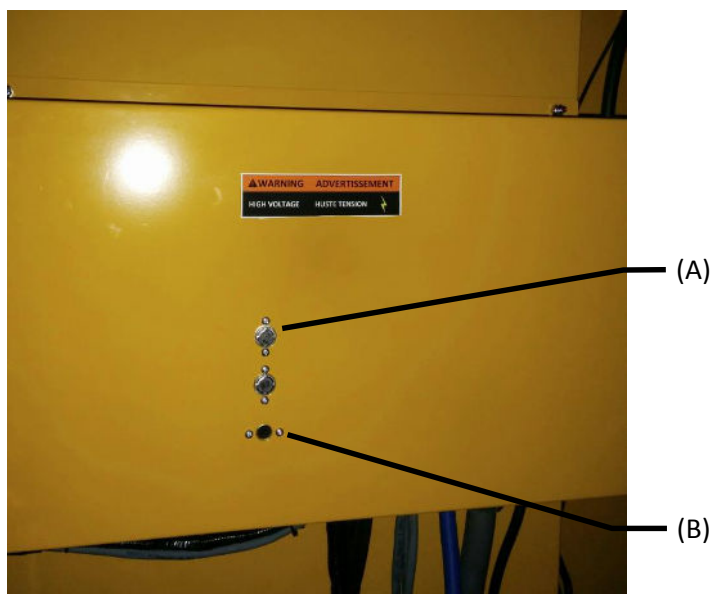
Figure 4. Rear of control panel (inside enclosure). Enclosure over-temp thermostat (A) and enclosure cooling fan thermostat (B)
